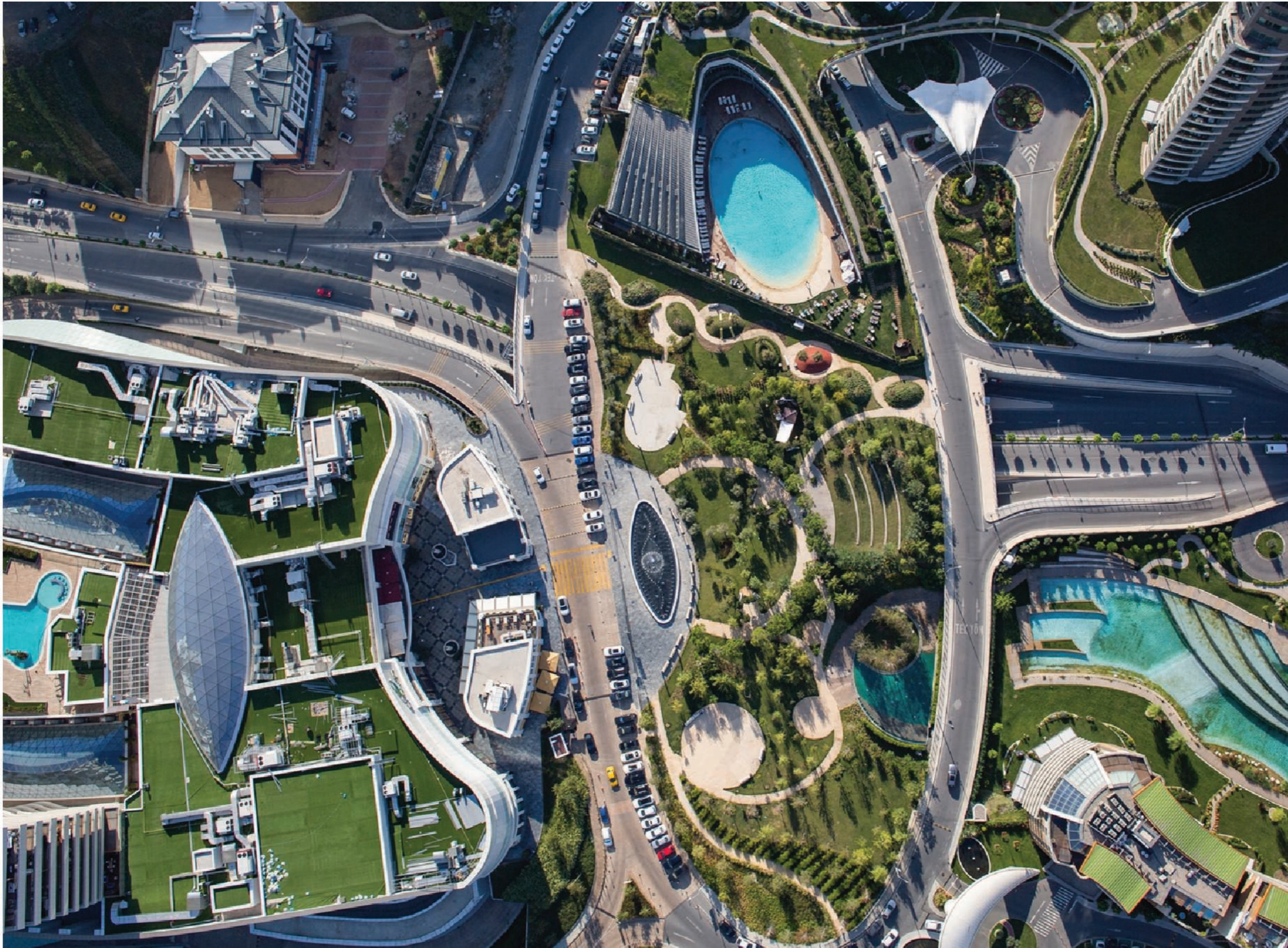
AKASYA COMPLEX EVRENOL ARCHITECTS
